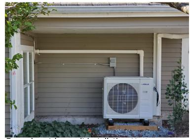
**Example outdoor unit installation:** Heat pump installed in an underutilized location with plenty of air flow. Unit is raised off the ground, level and with vibration pads on feet. White lineset covers match trim of building. Exterior to interior penetrations are weather protected (under eve) and appropriately sealed.
